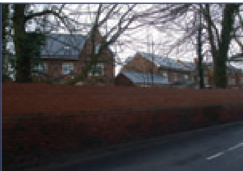
New development behind wall to Thorntree House, Middleton Lane
