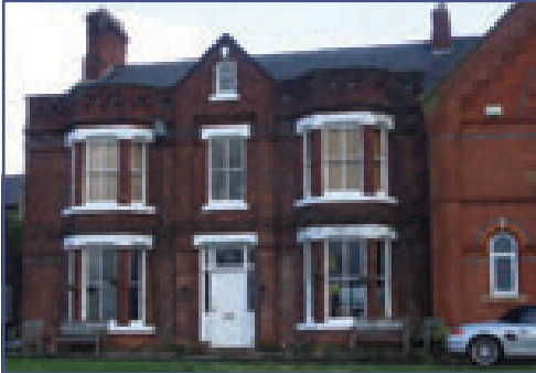
Traditional fenestration intact, no. 24 The Front
