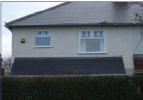
Weak, modern materials (windows & roof)
