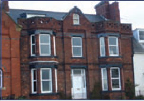
Loss of traditional fenestration, no. 25 The Front
