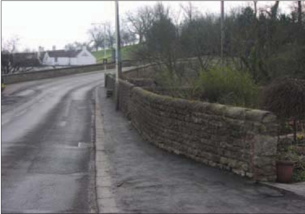
Image 1 – looking South towards Piercebridge Bridge, showing locally important stone walls
