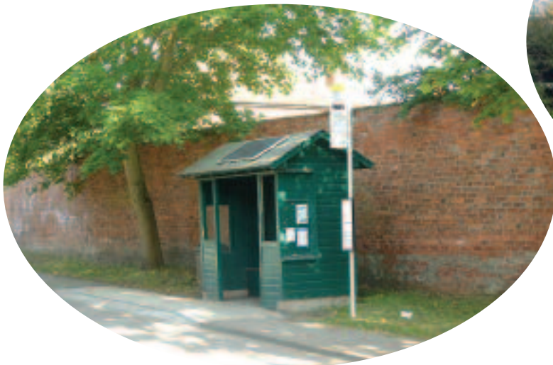
bus stop improvements in Hurworth
