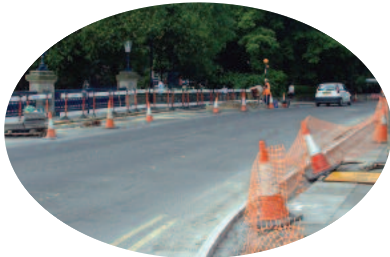
Preparatory works for Ring Road bus lane
