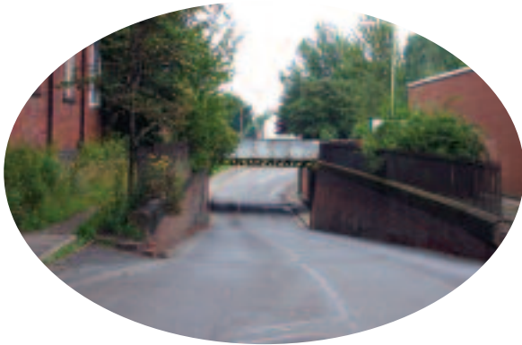
Cleveland Street before
