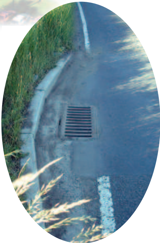
Gullies to address localised flooding
