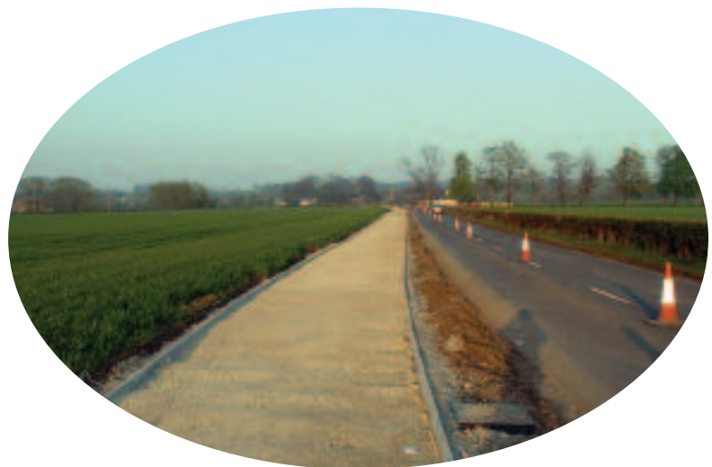
Hurworth, Neasham footway/cycleway under construction
