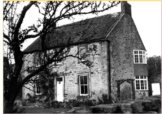
Image taken before unauthorised change of windows to uPVC.
