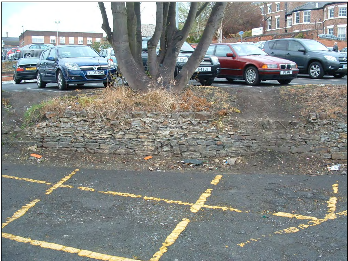
Figure 16: Low stone wall in car park west of Feethams, looking northwest
