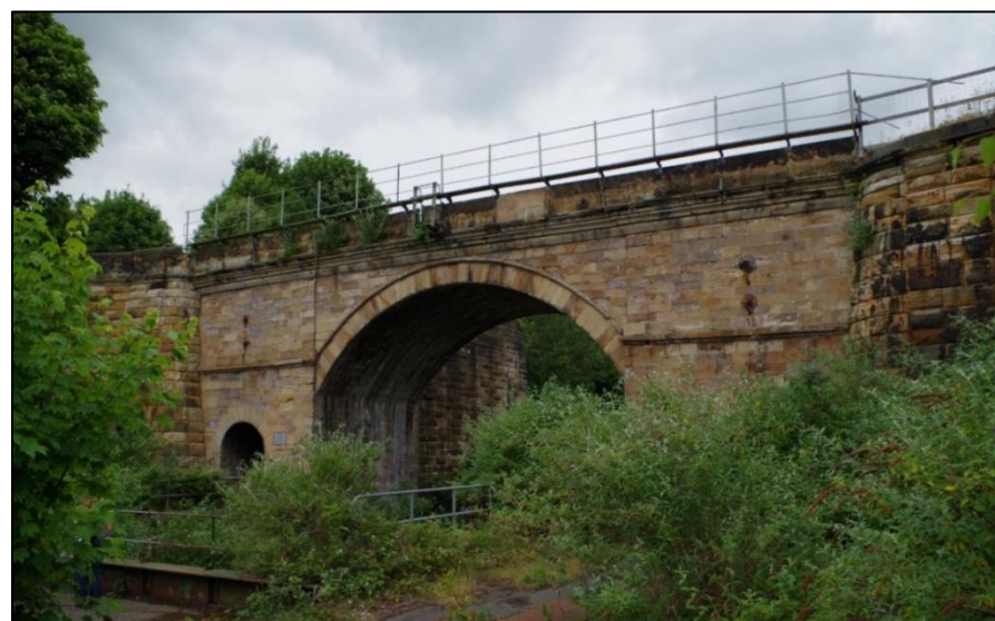
Plate 9. Skerne Bridge today viewed looking North-West
