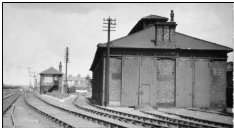
Plate 18. The Engine Shed looking north when it was still in use (courtesy of the Northern Echo)
