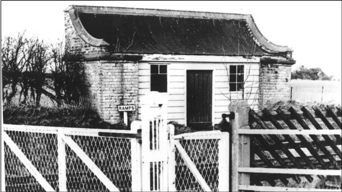
Plate 26. A waiting shed on the side of the S&DR line at Fighting Cocks c.1970. It was originally open fronted (Fawcett 2001, 127), but a new timber front applied when its use changed. Subsequent uses included a paraffin lamp shed and a toilet. The 'RAMPS' sign relates to the storage of ramps; always in pairs. They were 4ft long pieces of shaped metal which were laid beside the wheels of a derailed wagon – one ramp for the left wheels, one ramp for the right wheels. The wagon was then pushed up the ramps and back onto the tracks. 27 Some brick foundations and walling can still be seen on the site. (Photo John Proud Collection courtesy of Win Proud)
