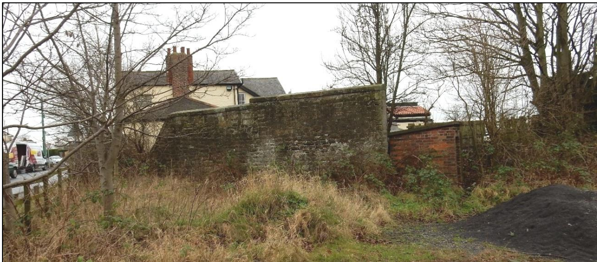
Plate 22. Some of the remains of the S&DR Coal Depot with the Fighting Cocks Inn beyond. A later signal box was located to the left of the wall.
