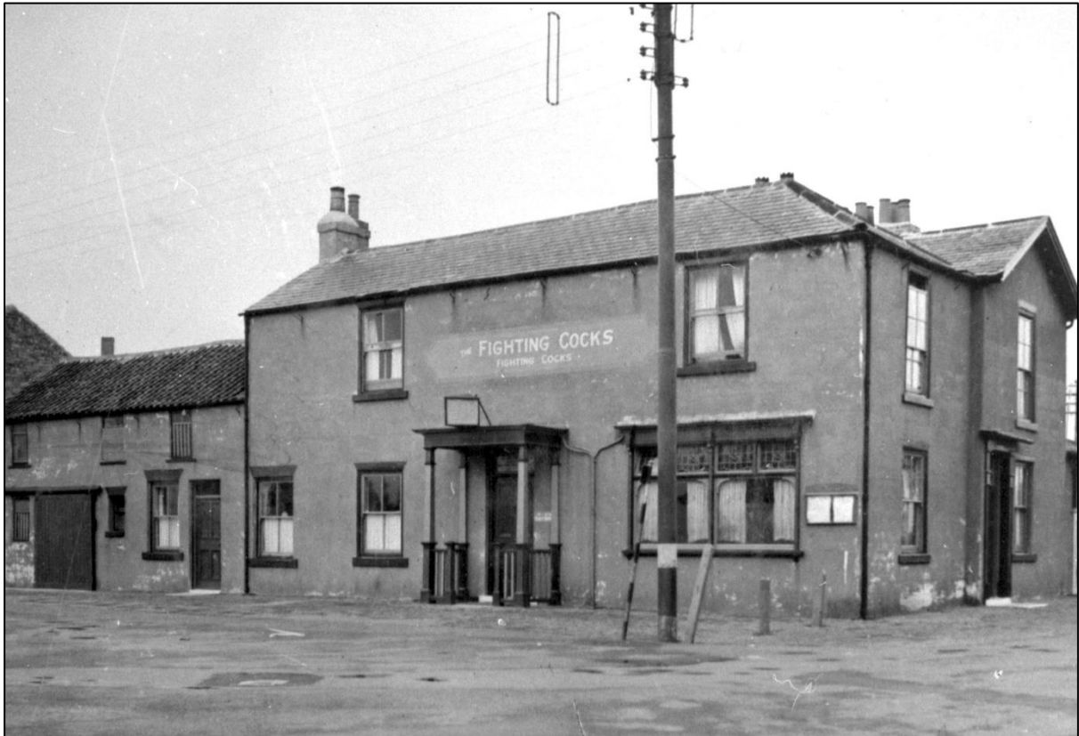
Plate 23. The Fighting Cocks Inn (undated image courtesy of Beamish Museum (NEG20016)). If the inn was built between 1823 and 1828 it would have had different fenestration detailing (multi pane windows) and smaller ground floor windows. The roofline was probably different too and the whole building originally smaller – it was extended in the late 19 th century.
