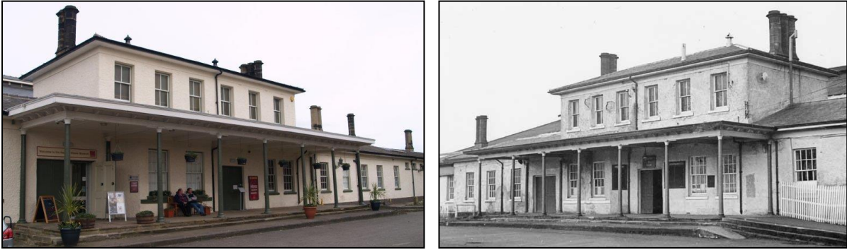
Plate 1. North Road Station 2016 (above right), and in 1972 (above right), prior to restoration and conversion to a museum.
