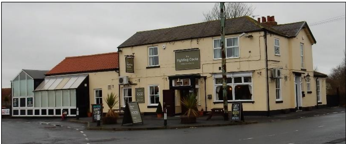
Plate 24. The Fighting Cocks Inn today. There is surprisingly little change from the undated image above. Presumably the render masks the blocked doorway to the left. The first floor window on the right has been enlarged and the replacement glazing is modern, but otherwise there are few alterations from the earlier photograph.
