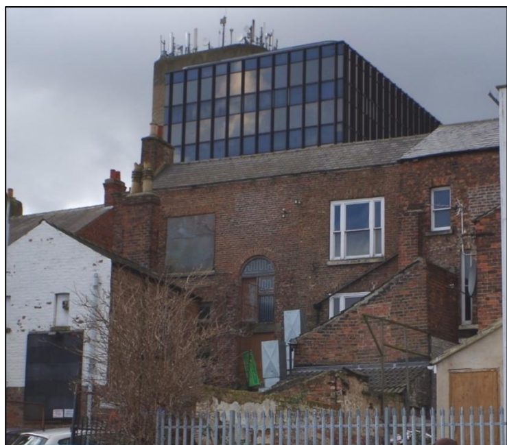
Plate 16. The back of Pease's house with the remains of a Georgian stair light window which once overlooked the fine gardens stretching down to the Skerne.
