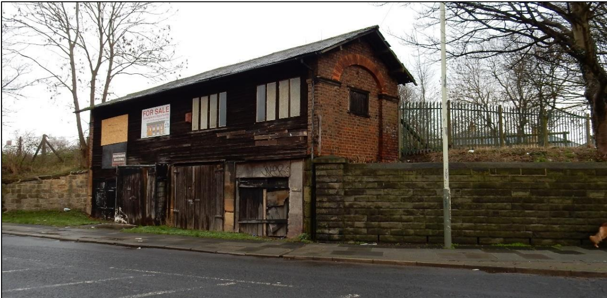
Plate 13. The Lime Depot. Waggons approached the building along the branch line from the left, passed through and dropped their loads through trap doors in the floor where the lime fell into bays. Builders could then purchase and collect lime from the ground floor level where carts could back up to the bays and then head back to where the lime was needed.
