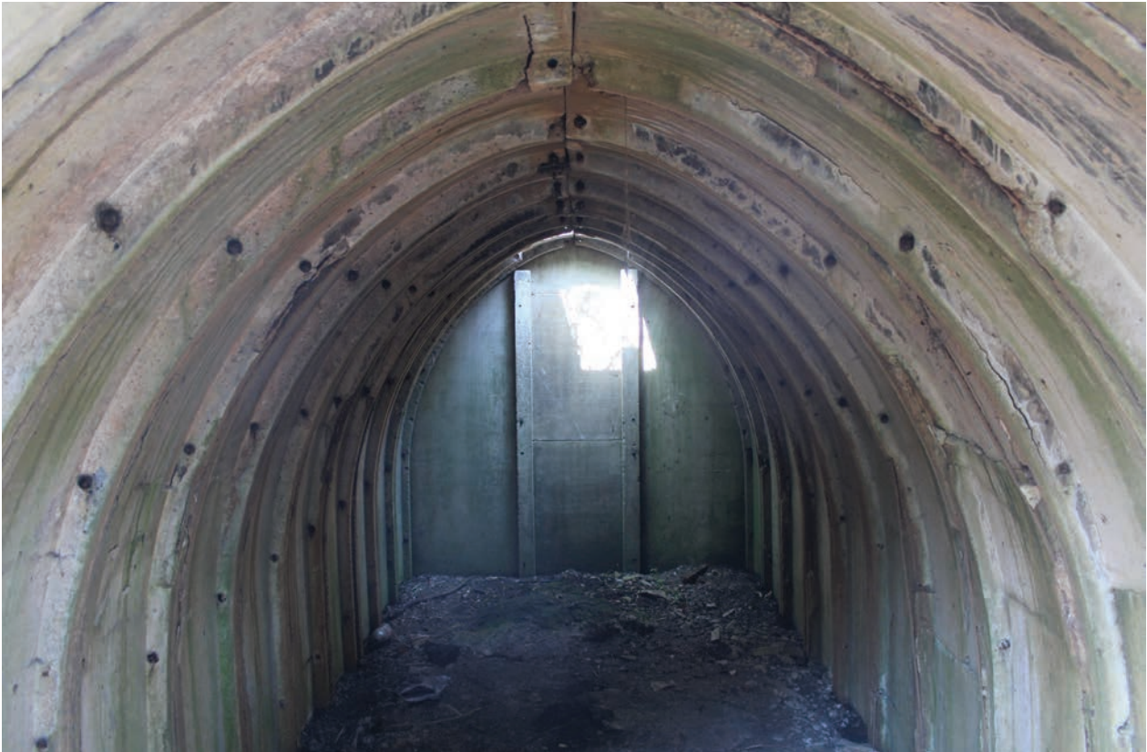
Figure 4.12 Interior of bunker, note ribbed vault concrete-cast ceiling
