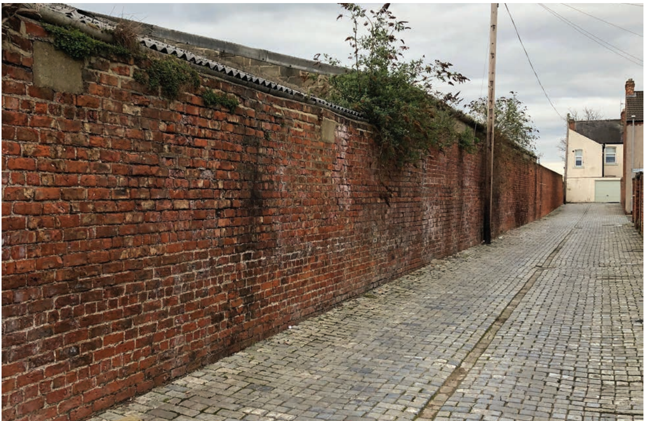
Figure 2.5 English-bond brick boundary at southern extent of the site
