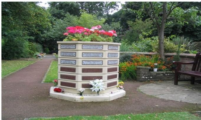
The memorial plaques are of red granite and are in relief lettering which ensures the plaque face will never deteriorate. Each plaque can accommodate three lines of text and is fixed to the planters using stainless steel screws.
