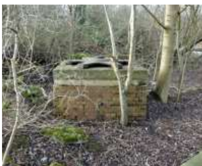
16 The crane base
