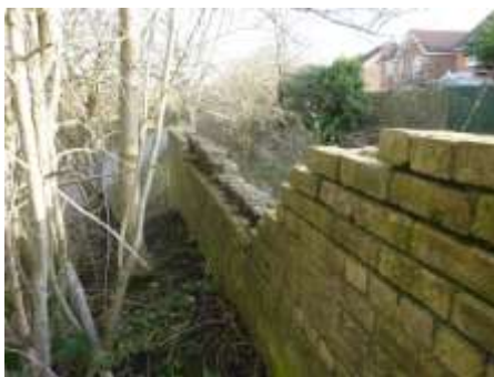
10 Old Mill wall; damaged eastern end
