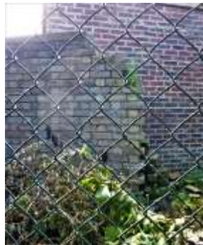
11 Old Mill wall; damaged western end
