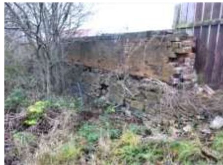
15 The retaining wall needing repair
