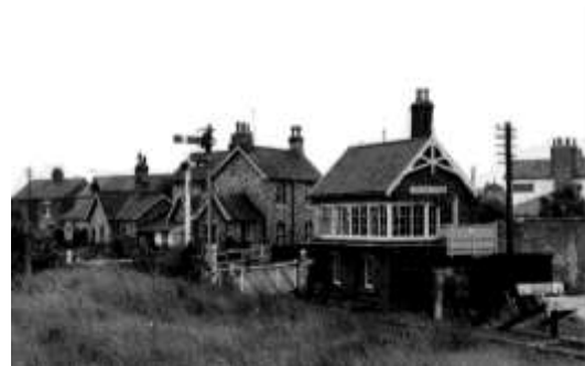
17 General view of the former crossing
