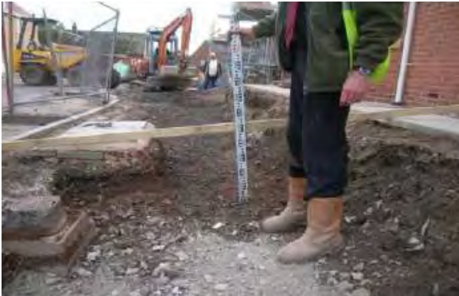
Photograph 3: Depth check of inert cover within areas of front gardens.
