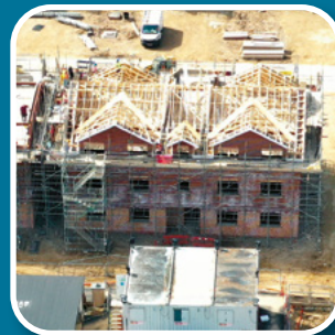
ALLINGTON WAY PROGRESS
