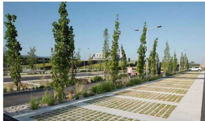
Example showing how grass crete and soft landscaping can be used to soften car parking and provide a permeable surface
