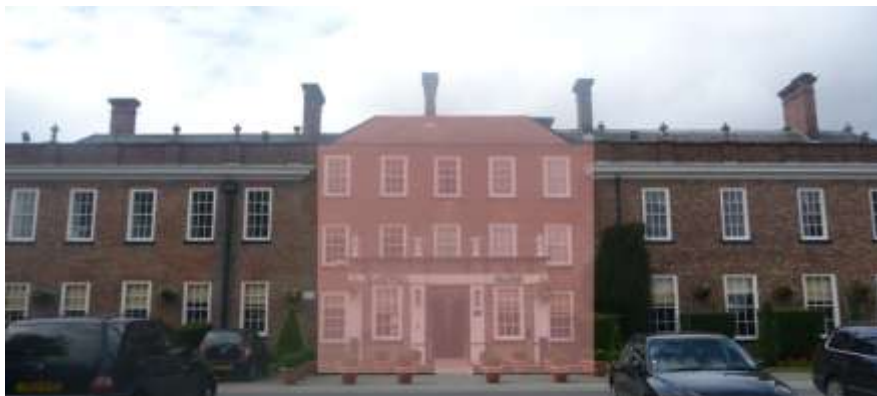
Plate 1. The central bay, minus the later porch, (shaded) represents the earliest part of the house and would have been the elevation seen on the approach to the house from the main entrance through the formal grounds from 1710
