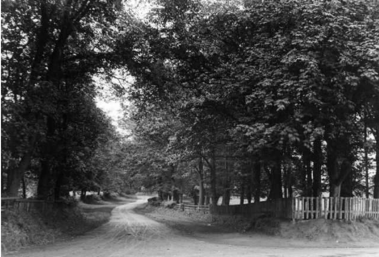
Plate 9. Blands Corner Lane End in c.1900. The new extended southern boundary of the park was defined by rustic wooden fencing mirrored on the Blackwell Hall side of the road. This remains the predominant fencing type on Carmel Road South, although the presence of advertising banners today does little to enhance to historic character of the area
