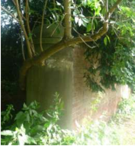
Plate 4. One of the stone gateposts that marked the Grange access points off Blackwell Lane
