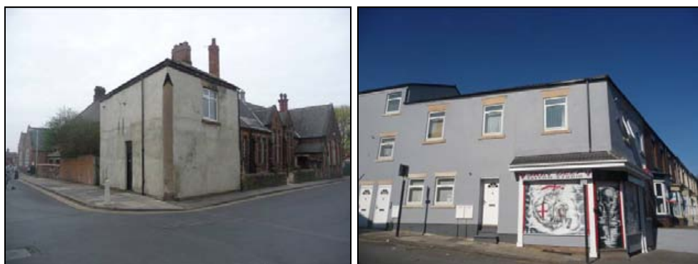
Plate 9. Cement renders damage the brickwork beneath, reduce thermal performance, cause condensation and damp and create a negative visual impact.
