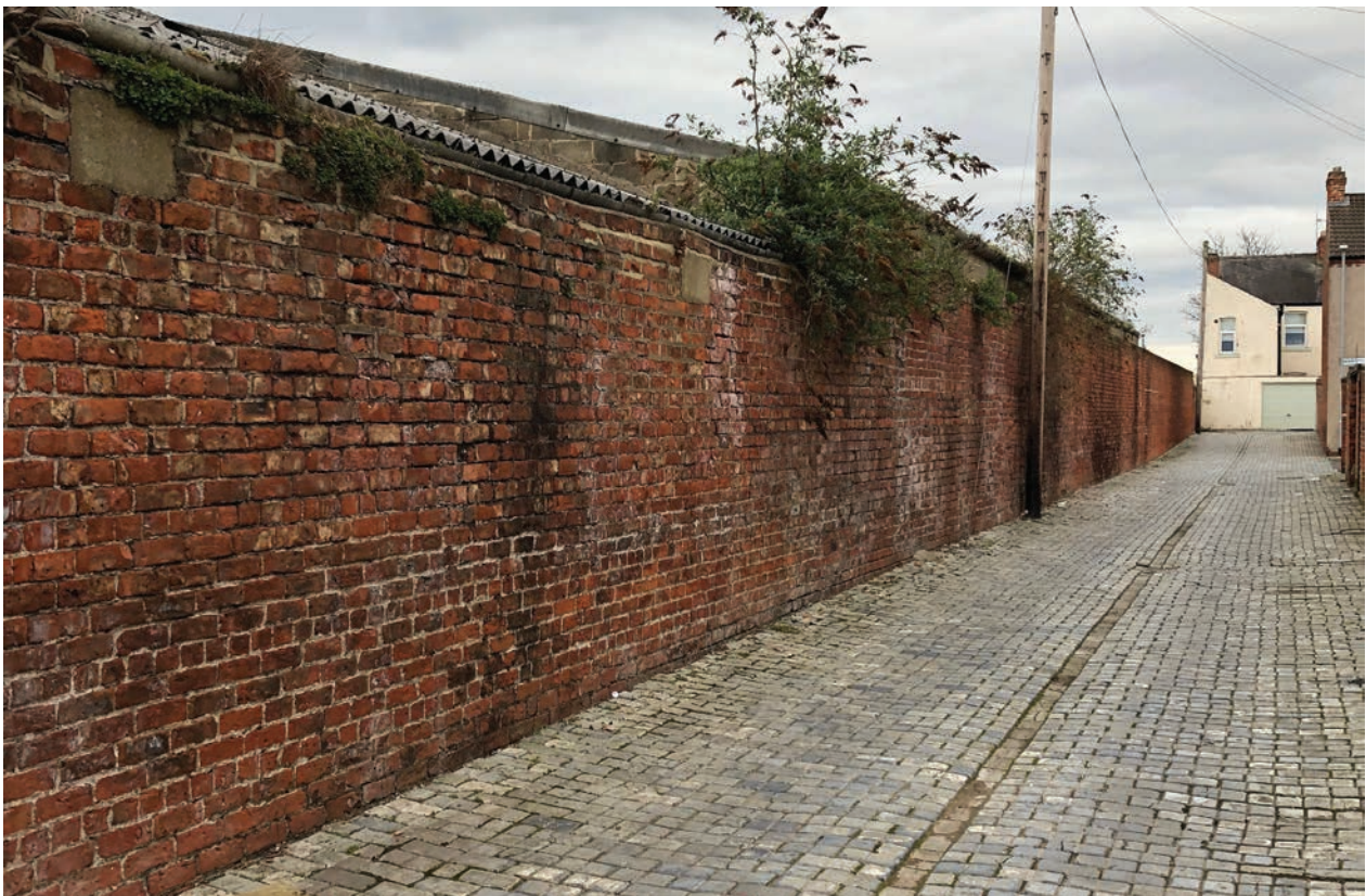
Figure 2.5 English-bond brick boundary at southern extent of the site
