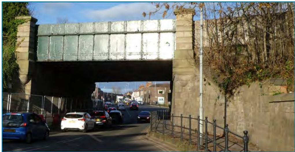
[6] Railway Viaduct (photo © Gaby Rose, 2023): Plans to build a bridge were begun in the 1840s, and the bridge finally built in 1856; altered/rebuilt in 1876, and road level further dropped after 1949 to allow for double-decker busses 103 . An early photograph shows a plaque with the date MDCCCLVI on the side. Altered prior to 1935.
