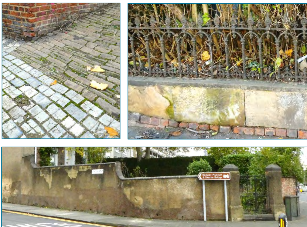
Top left: Back lane with scoria and sandstone block surfacing. Top right: Ornate, cast-iron railings on top of ashlar stone/brick boundary walling between private front garden and public realm. Bottom: Rendered garden wall on street corner with stone copings and prominent gate piers. (Photos © Gaby Rose, November 2023)
