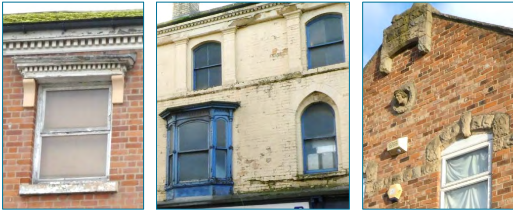
Left: Brick building with Italianate stone detailing to eaves and canopy above window. Centre: [E] Livingstone Building – All walling and detailing in brick, later painted; decorative bay window constructed in timber. Right: [F] 1 Leadenhall Street – Distinctive stone carvings by Robert Borrowdale (Photos © Gaby Rose, November 2023)
