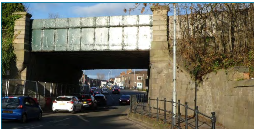
[6] Railway Viaduct (photo © Gaby Rose, November 2023): Plans to build the bridge had begun in the 1840s. It was finally built in 1856, altered/rebuilt in 1876, and the road level further dropped after 1949 to allow for double-decker busses 107 . An early photograph shows a plaque with the date MDCCCLVI on the side. Altered prior to 1935.
