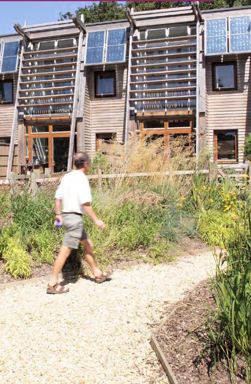
*Low energy housing with passive solar design, including shading to prevent overheating in summer, and highly insulated thermal mass construction.*
